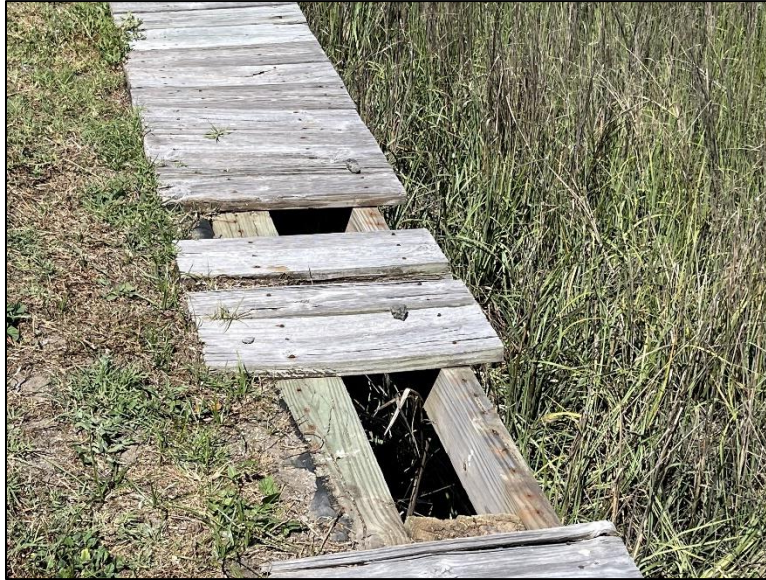
Figure 3.14. Missing Decking
