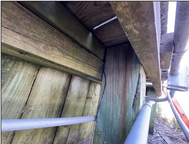
Figure 3.3. Split Top Waler Near West End of Bulkhead
