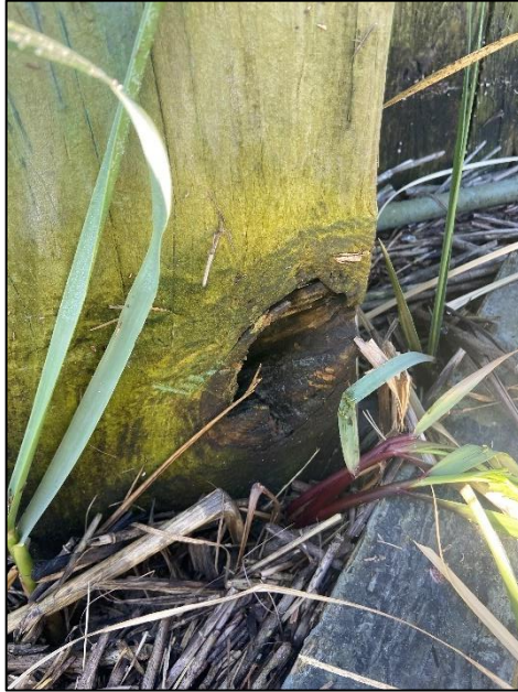
Figure 3.8. Knot in Third Pile from Pier
