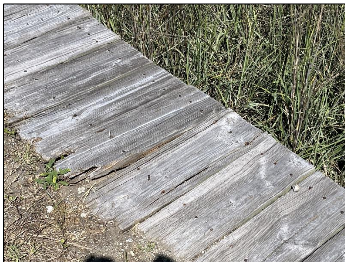
Figure 3.13. Deteriorated Decking
