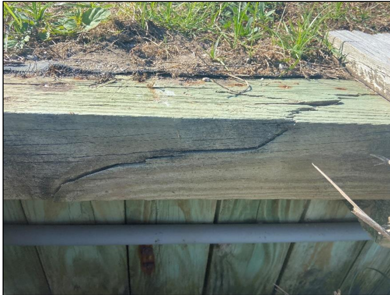
Figure 3.4. Split Top Waler Along West End of Bulkhead
