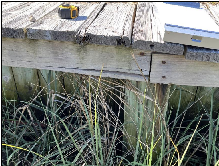
Figure 3.5. Split 3x6 Front Nailer Near Middle of Western Section of Bulkhead
