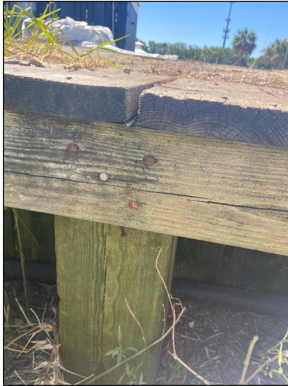
Figure 3.6. Split 3x6 Front Nailer Near Eastern End of Bulkhead
