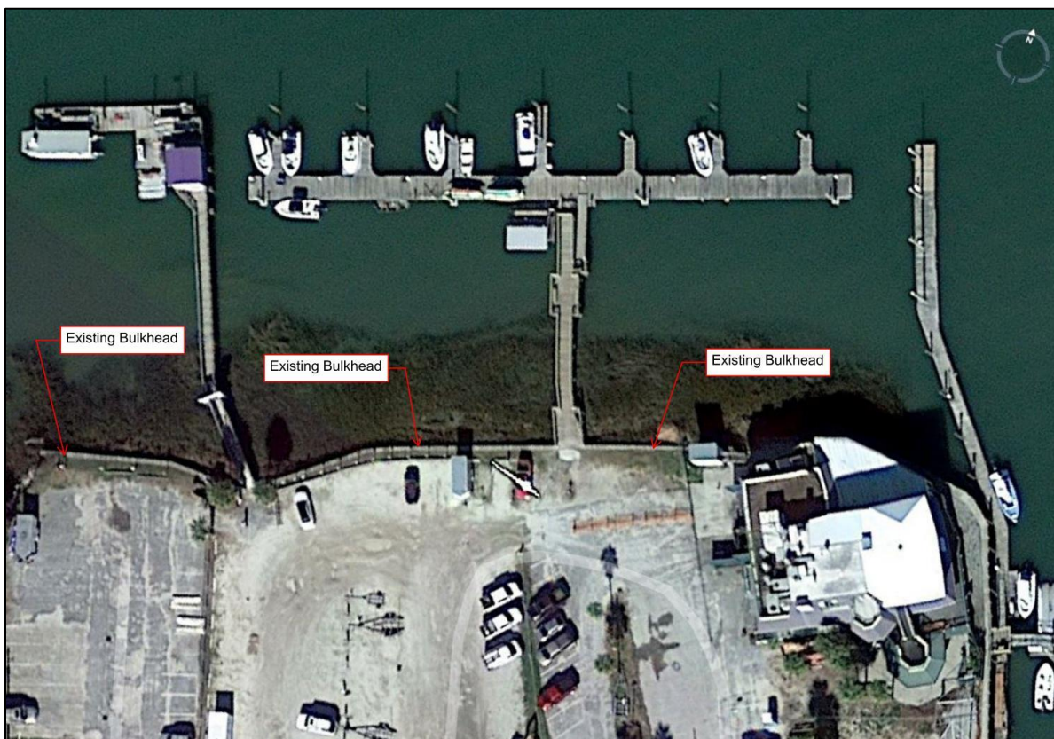
Figure 2.1. Aerial Showing Existing Bulkhead
