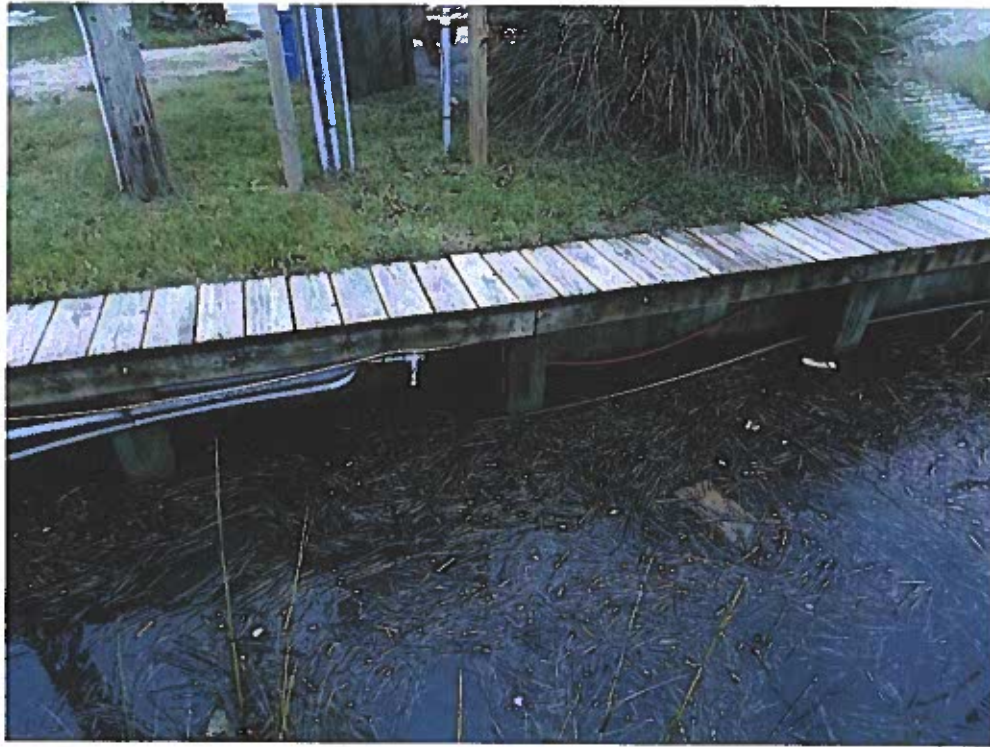
Typical Timber Bulkhead along Intracoastal Waterway
