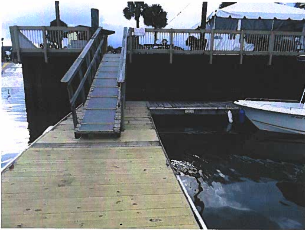
Gangway Landing and Re-Decked Dock Section
