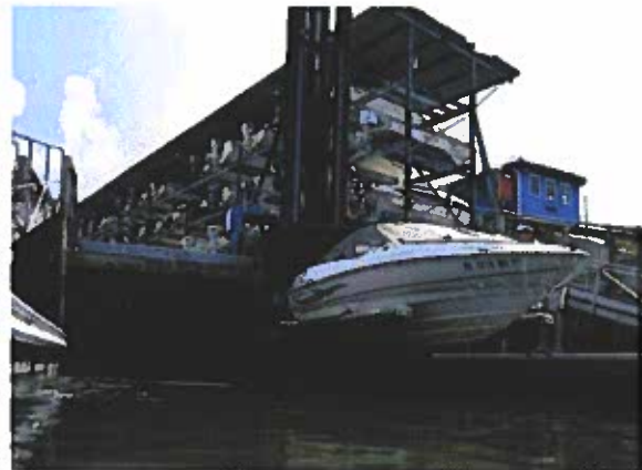
Shem Creek Marina Drystack Facility
