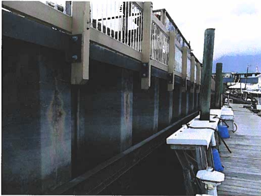
Steel Sheet Pile Bulkhead
