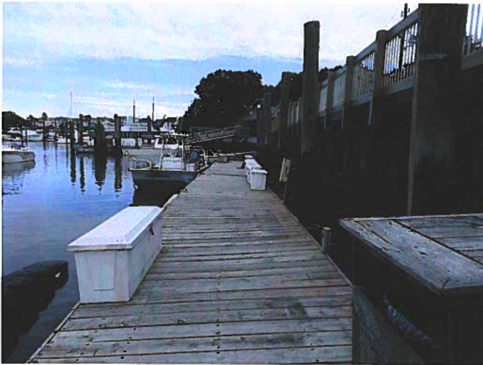
Shore-Side Floating Dock (Note: wave in framing)
