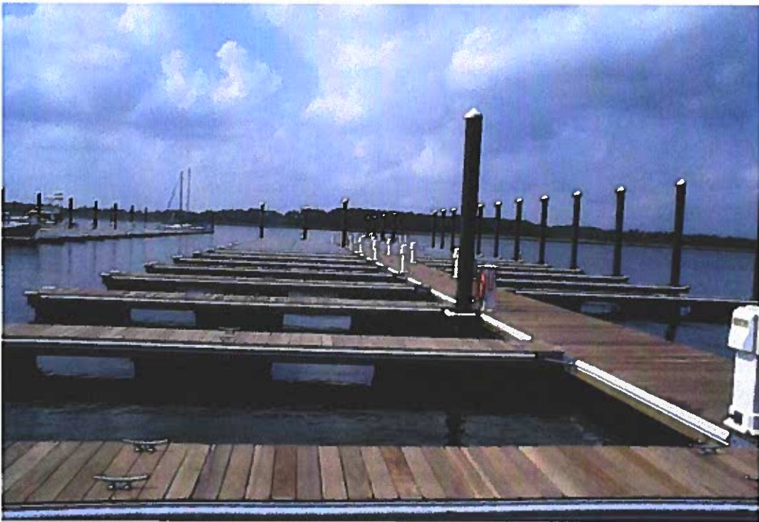
Timber Frame Floating Dock with Ipe Hardwood Decking
