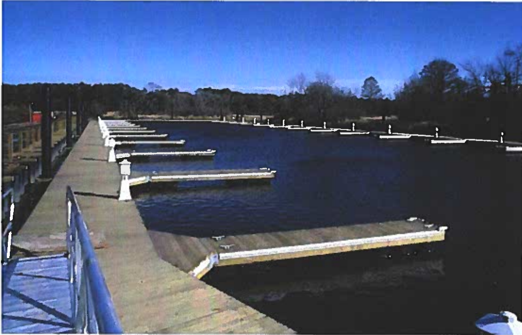
Floating Timber Docks with Southern Yellow Pine Decking
