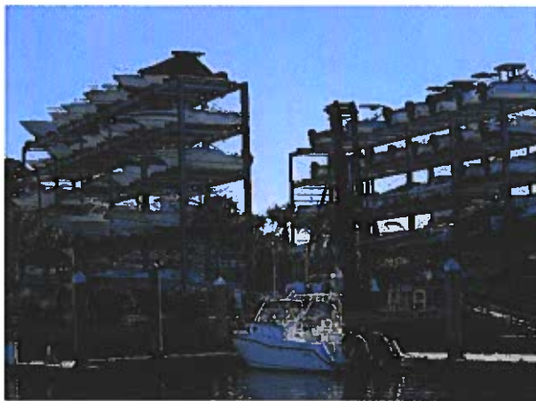
Open, Uncovered Racks at Ripley Light Marina & Drystack
