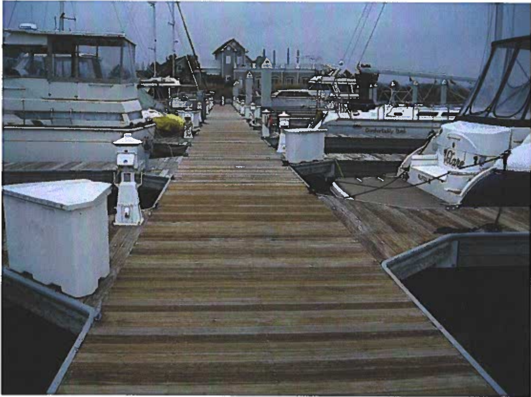
Aluminum Frame Floating Docks with Ipe Decking
