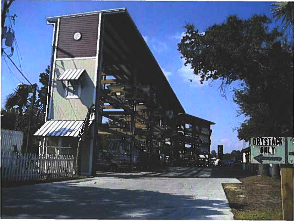
Three-Sided Drystack Storage Building (Magwood Marina, Old Village, Mt. Pleasant)
