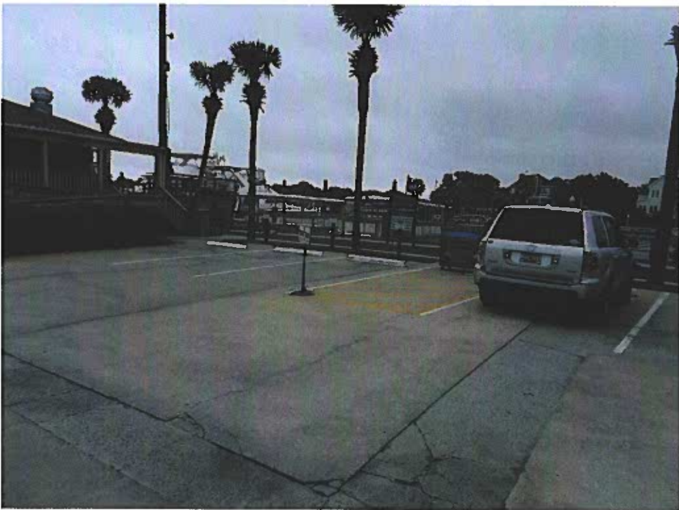
Concrete Parking Area
