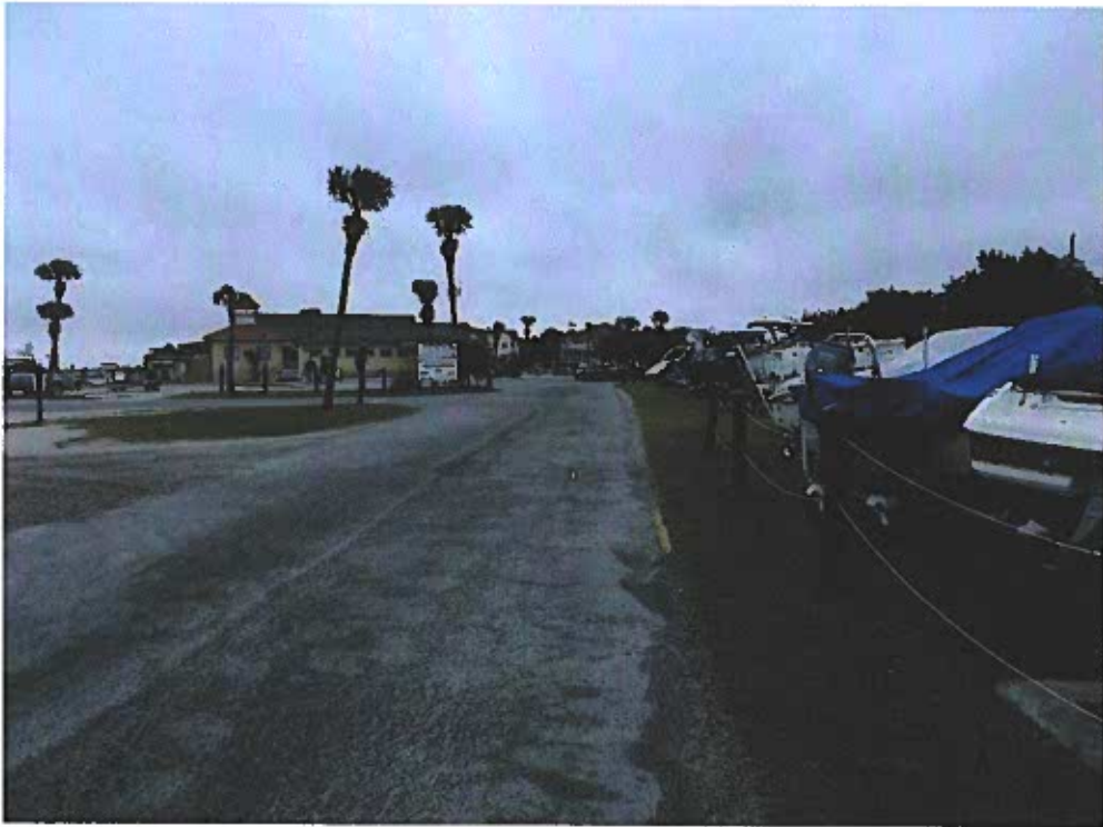
Main Entrance – Asphalt Paving
