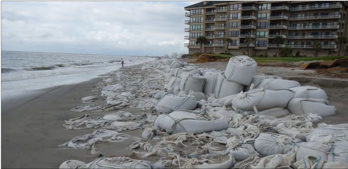
FIGURE 2.5. To prevent additional erosion, sandbags were installed along several structures from Shipwatch to Ocean Club from 2004 to 2007.
