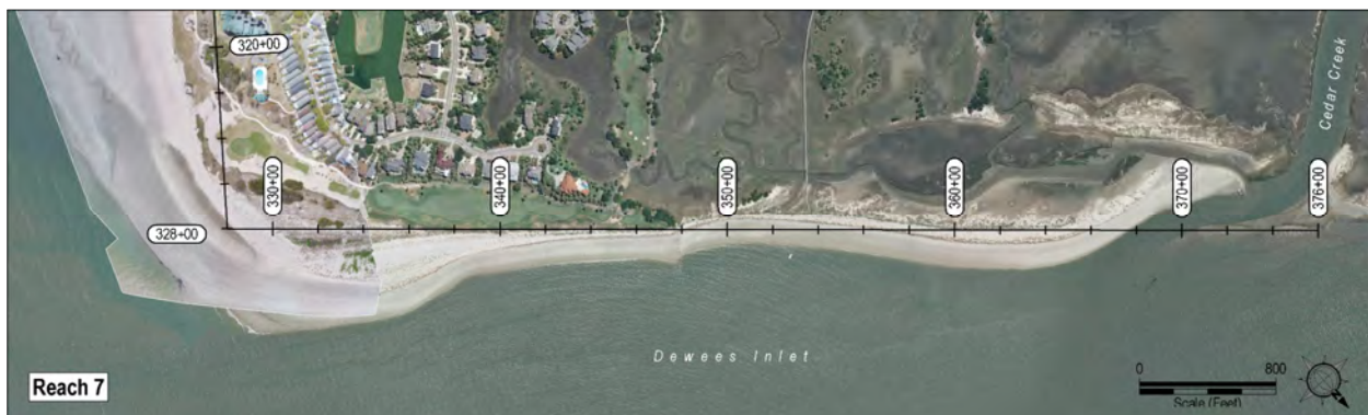
FIGURE 4.4. Baseline stationing along Reach 7 encompassing the length of beach between lines 330 and 370.
