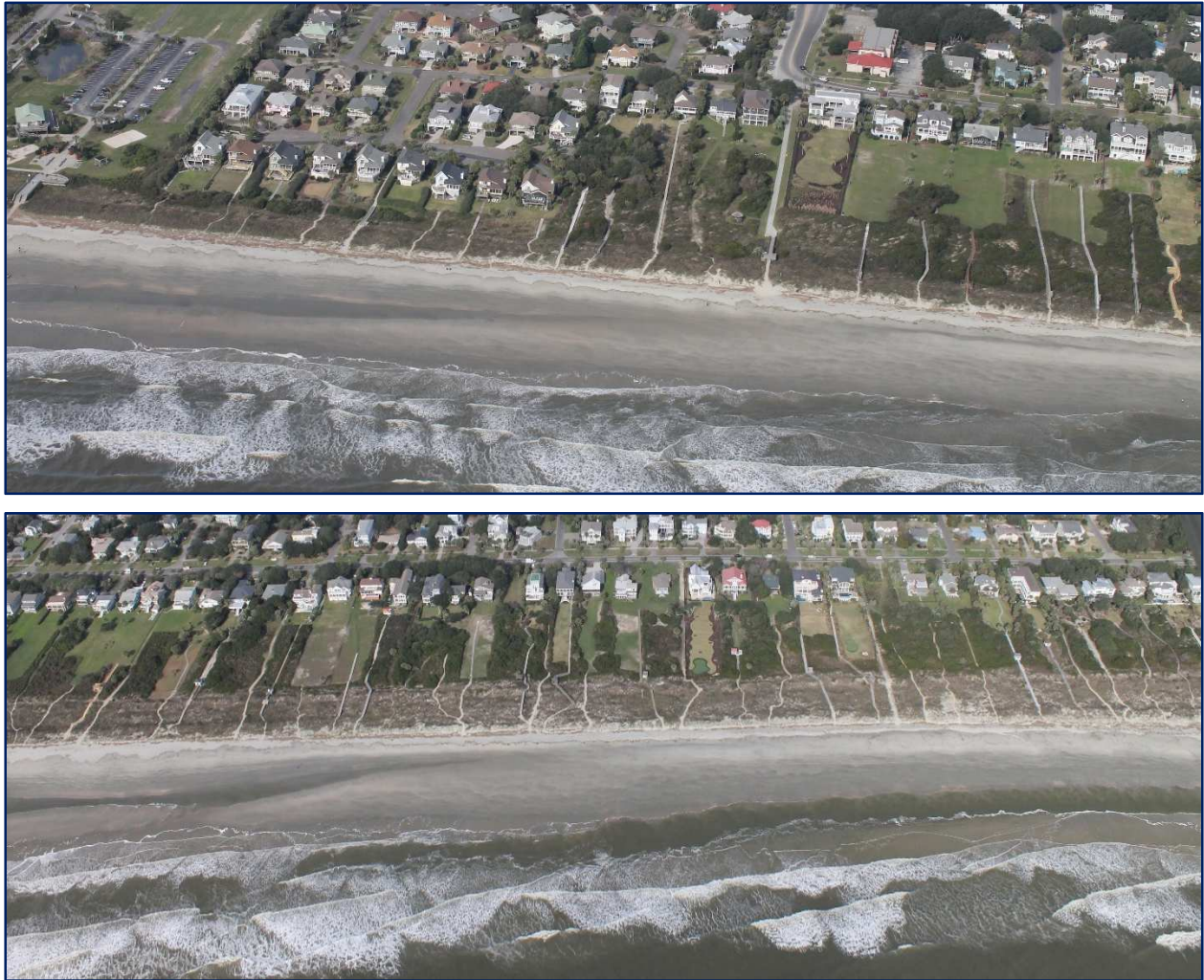
FIGURE 3.35. January 2016 aerial images of Reach 3. [UPPER] The area from the County Park to 22 nd Avenue. [LOWER] Area between 27 th Avenue and 33 rd Avenue.
