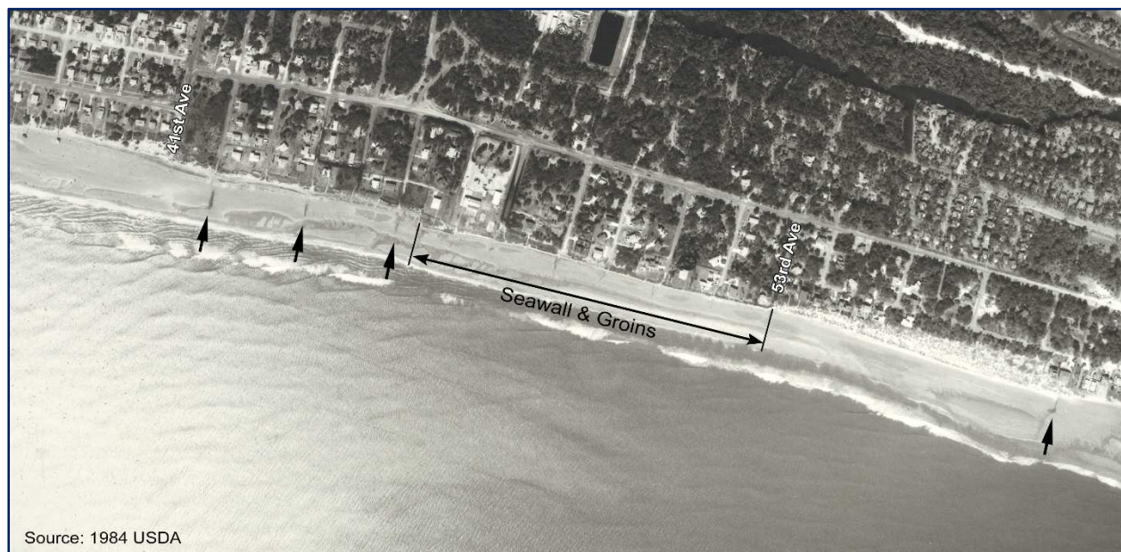
FIGURE 1.4. 1984 aerial image of Isle of Palms between 39th Avenue and 57th Avenue showing groins and a seawall installed along the beach. Groins are indicated by the arrows.
