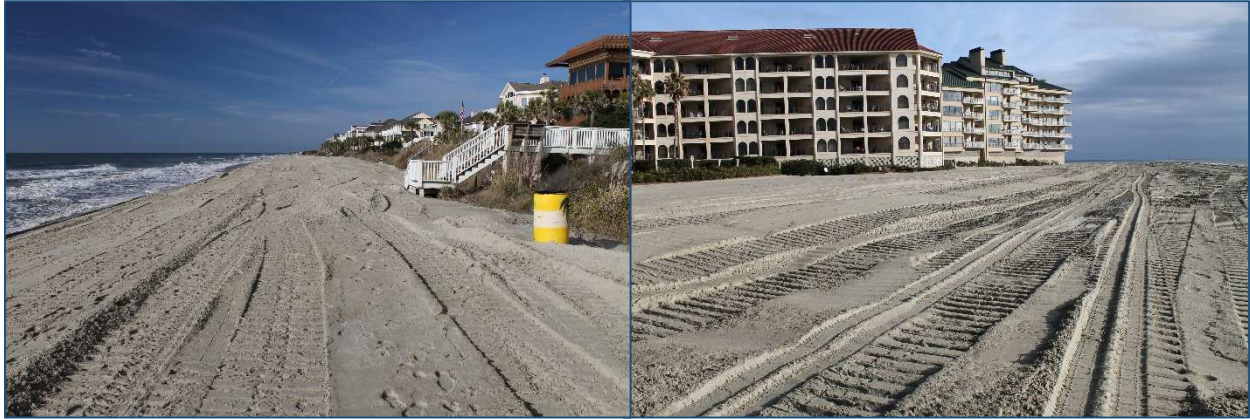
FIGURE 1.7. Post-construction photos of the 2014–2015 shoal management project. [LEFT] The area fronting Dunecrest Lane. [RIGHT] The area fronting Seascape and Ocean Club.
