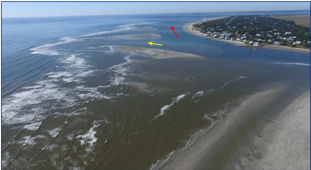
FIGURE 3.9. October 2015 aerial image of Breach Inlet. Arrows show the main (adjacent to Sullivan's Island) and secondary channels.
