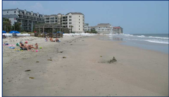
FIGURE 3.17. Sandbags were installed in front of most of the condominium units prior to the 2008 restoration project.
