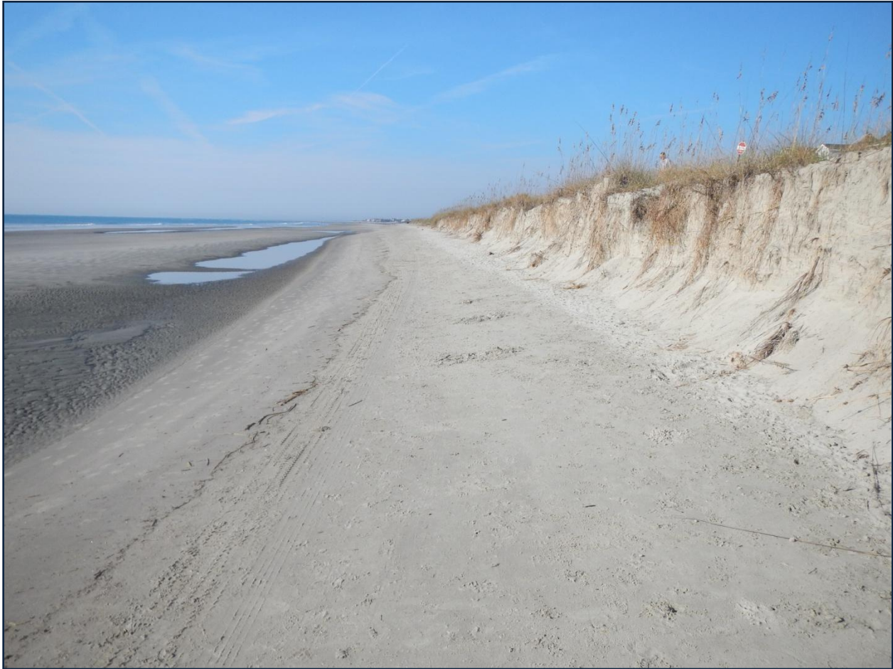
Looking west from Station 50+00 (near 7 th Ave). This was the only area showing an active escarpment in October 2013. There was a small erosional arc centered at this station.
