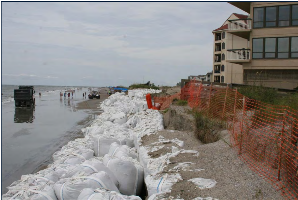
FIGURE 3.41. July 2013 photo of the temporary sandbag revetment placed by property owners along the critically eroded portion of Wild Dunes.
