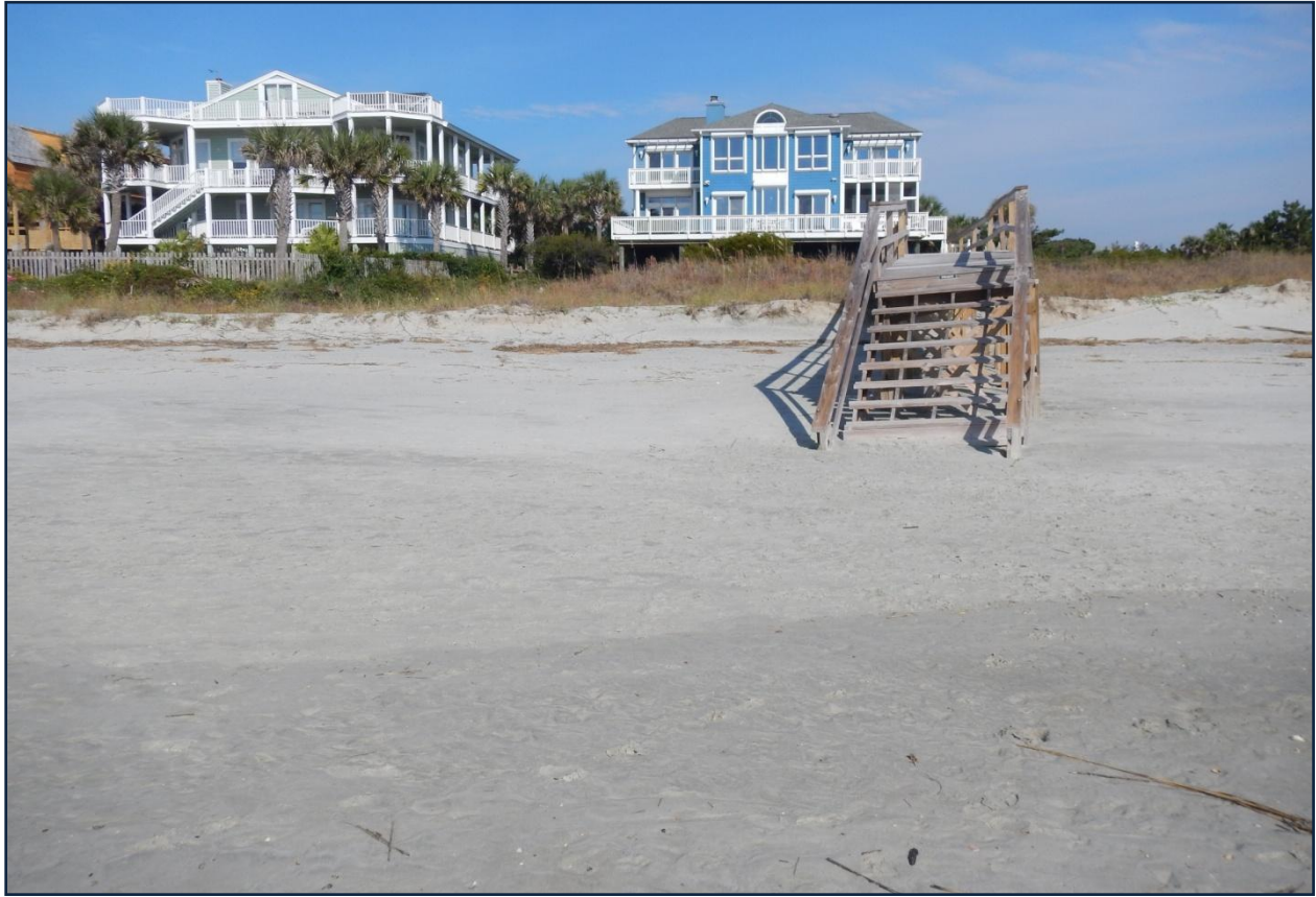
Landward view at station 12+00 showing low dunes lacking sufficient elevation to offer significant storm protection. This area had eroded heavily from July 2012 to July 2013 but was accretional from July 2013 to October 2013.
