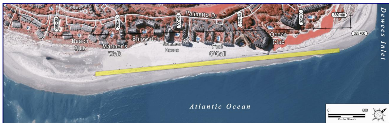
FIGURE 3.8. Reach 6 spans from the Wild Dunes Property Owners Beach House (station 280+00) to the 18 th fairway of the Wild Dunes Links Course (station 328+00). The approximate limits of nourishment Reach B are identified by the yellow bar. March 2009 aerial image by Independent Mapping Consultants Inc.
