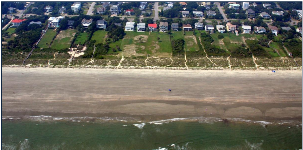
FIGURE 3.25. Aerial views along 27 th Avenue to 30 th Avenue (upper) and 25 th Avenue to 29 th Avenue (lower) after passage of Hurricane Irene in August 2011.
