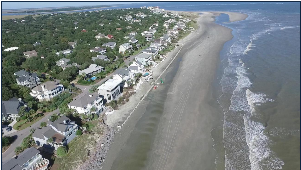
FIGURE 6. October 2015 post-storm aerial images of the area near the Grand Pavilion (upper) and Beachwood East (lower). The Grand Pavilion walkover is in the foreground of the upper image. This area experienced the most dune erosion and volume loss during the storm. The experimental wave dissipation device along Beachwood East was damaged during the storm. Houses here have installed sandbags and have little-to-no, dry-sand beach fronting the structures.
