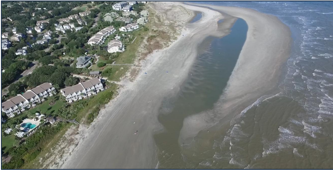
FIGURE 10. October 2015 post-storm aerial image of the attaching shoal along Wild Dunes community. The western edge of the shoal remains unattached (lower portion of image), while the eastern edge is attached. Transferring sand from the attached shoal to the eroded areas would be beneficial to facilitate additional merging of the shoal sand.
