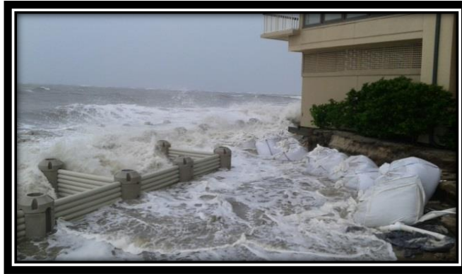
Building One at Ocean Club is protected by both sand bags and a wave dissipation system
