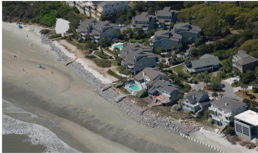
Figure 21. April 5, 2016 photo of exposed rock revetment near Seagrove/Beachwood East.
