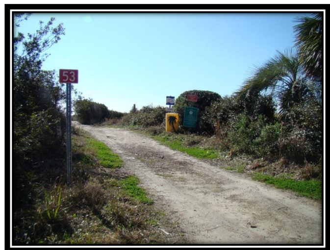
Example of one of the City's emergency vehicle accesses
