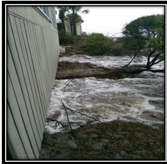
Ocean washing under home on Beachwood East
