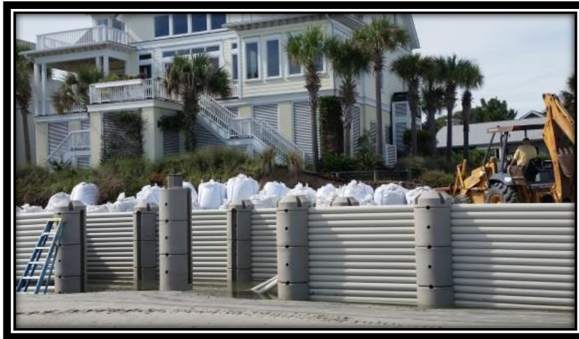
Sandbags being added landward of a wave dissipation system
