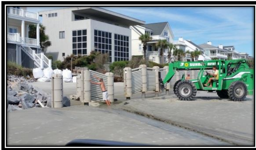
Repairs to a wave dissipation system following a high tide
