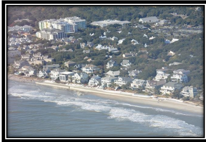
Wave Dissipation Device at Beachwood East on Isle of Palms
