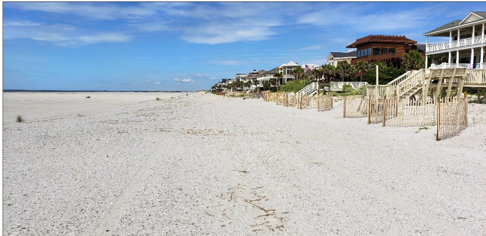
FIGURE 4.16. Ground photos of Reach 6. There remains a low swale on the landward side of the berm, seaward of the pre-project dune line.
