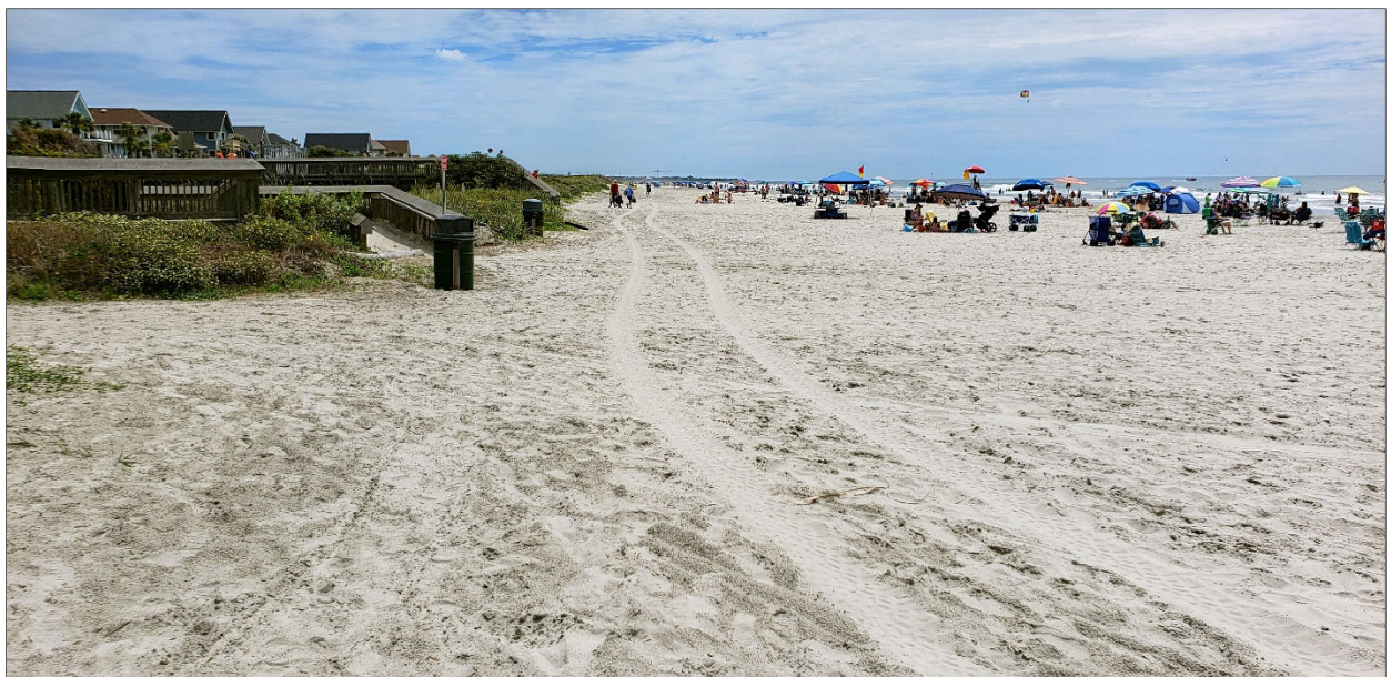
FIGURE 4.23. The long-term trend for Reach 3 is stable to accretional. Dwellings in the reach are generally set back from the beach between 400 ft and 500 ft.
