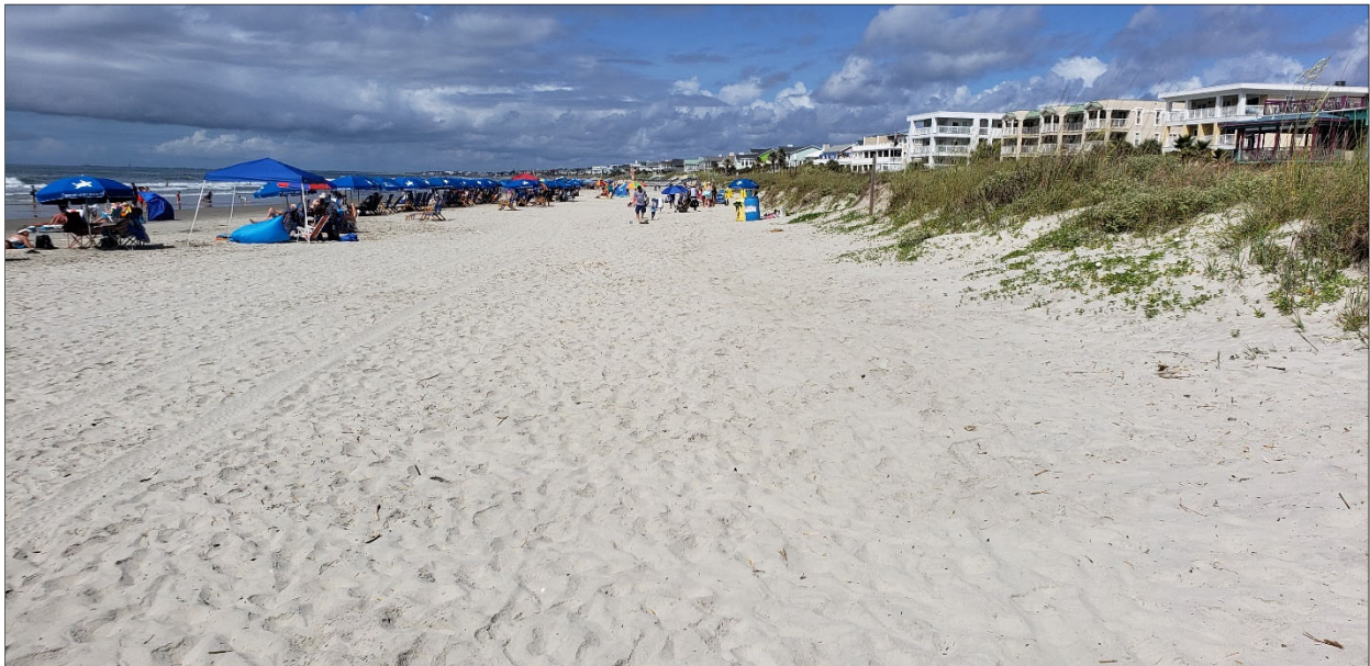
FIGURE 4.27. Compared to the 2009 condition, the eastern half of the reach has accreted while the western half has eroded. [UPPER] The healthier condition of the eastern end of the reach (south of the pier). [LOWER] Western end which is undergoing a higher rate of erosion.
