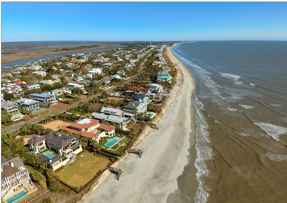
FIGURE 4.31. Aerial photos taken in December 2019 show that most of the dune constructed following Hurricane Irma remained in place north of 2nd Ave, but was mostly eroded west of Station 20+00.
