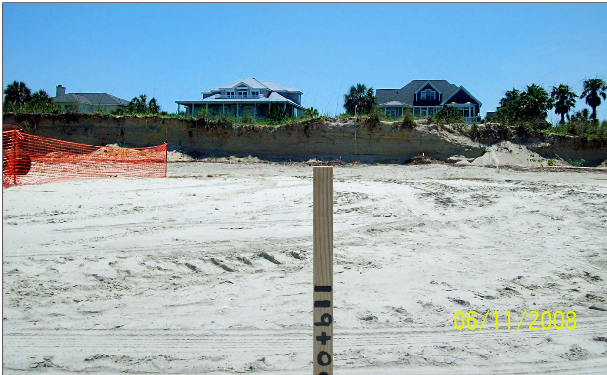
FIGURE 4.5. In 2008, a significant erosional escarpment was documented along most of Reach 7 seaward of the 17 th tee box of the Links Course.
