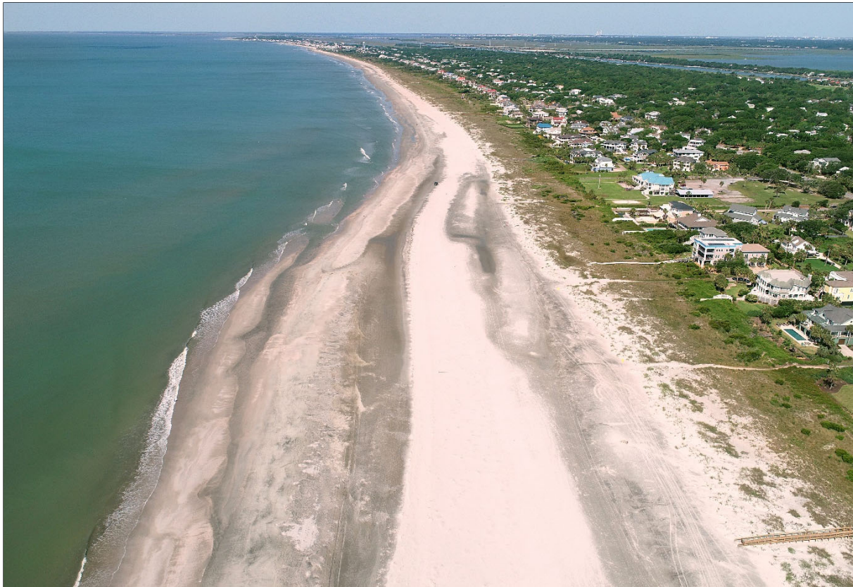
FIGURE 4.19. By being positioned downdrift of the nourishment area, Reach 4 receives nourishment sand spreading from the placement area as well as spreading shoal sand. This reach has gained sand every year since 2009 except 2016.
