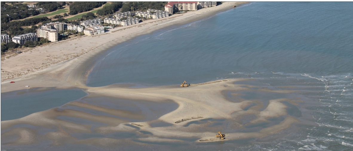
FIGURE 2.10. January 2015 aerial image of the 2014–2015 shoal management project showing equipment transferring sand from an attaching shoal to the eroded beach.
