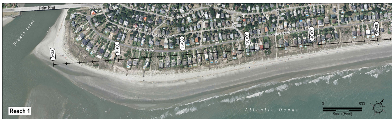
FIGURE 4.27. Baseline stationing along Reach 1 which encompasses the beach between Breach Inlet and 6 th Avenue.
