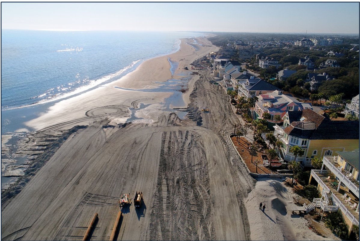
PHOTO 8. Aerial photograph taken from CSE's drone overlooking beach building operations in front of Beachwood East on 21 January 2018.
