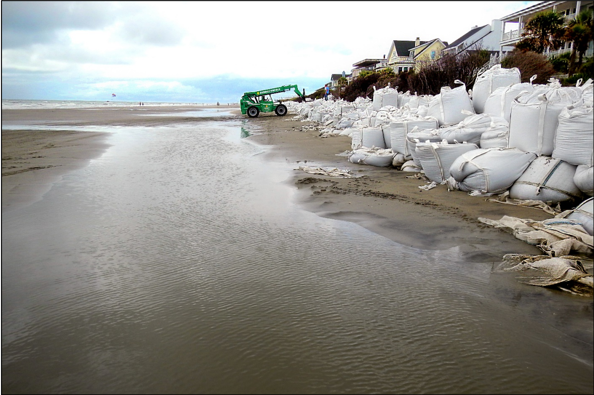
PHOTO 19. Looking south at Beachwood East back in 2014 during sandbag installation.
