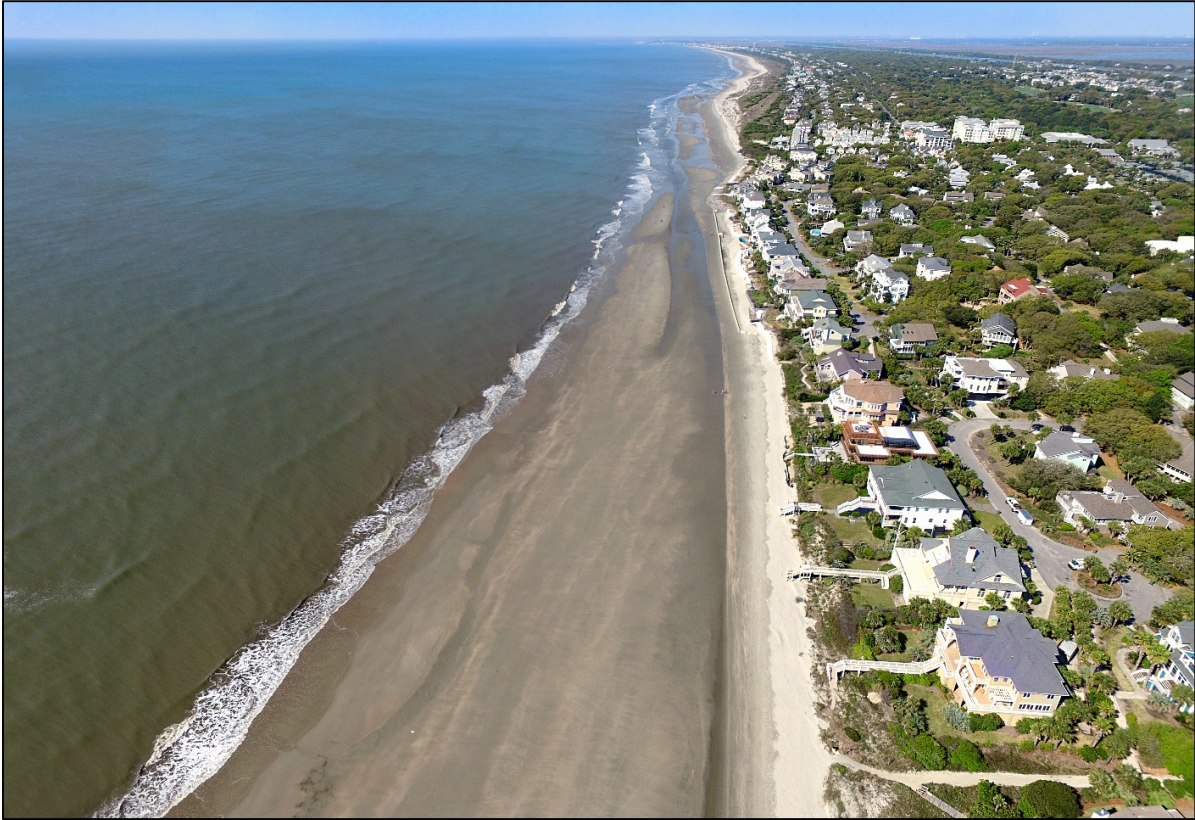
PHOTO 17. Pre project look at Reach 1 (Stations 236+00 through 280+00) with Wave Dissipation System in front of houses at Beachwood East.
