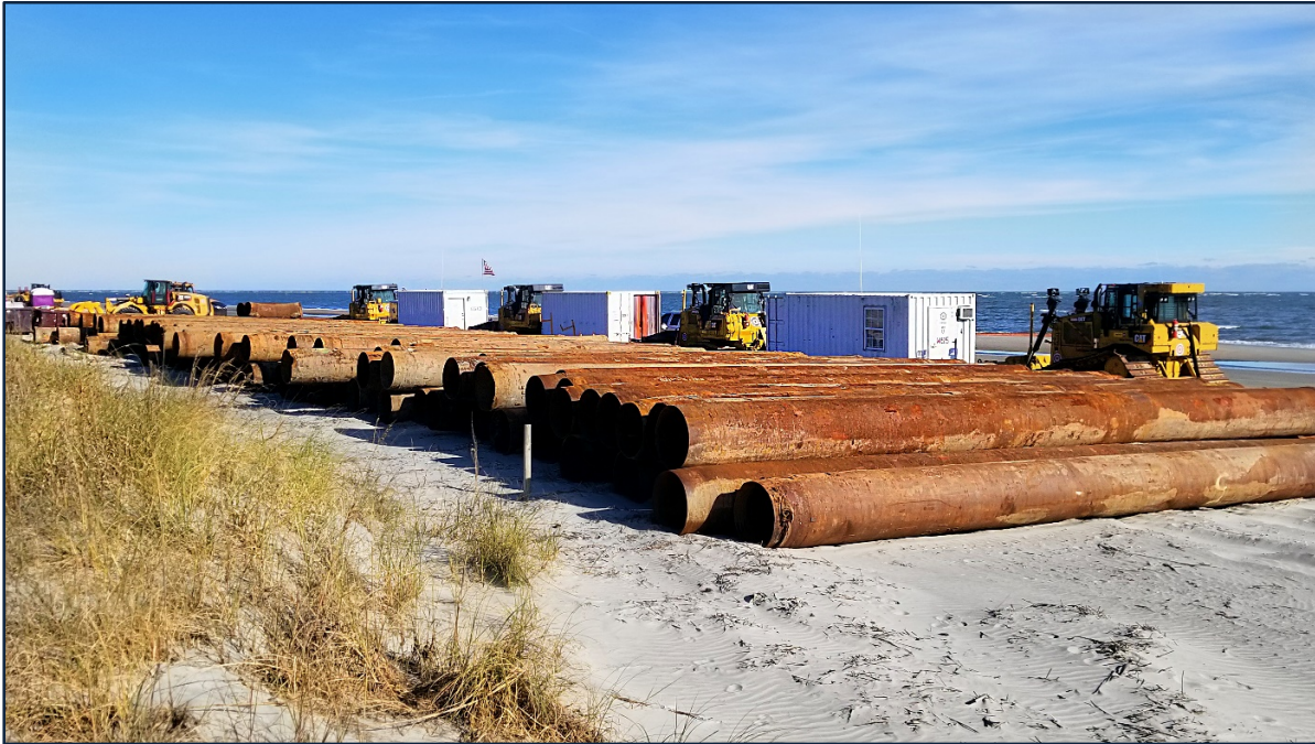
PHOTO 1. Shore pipe and equipment staged and ready to start construction.
