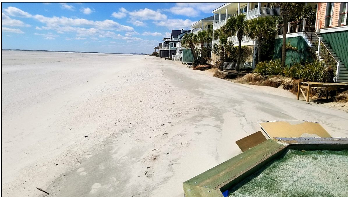
PHOTO 20. Beachwood East in March 2018 after construction.
