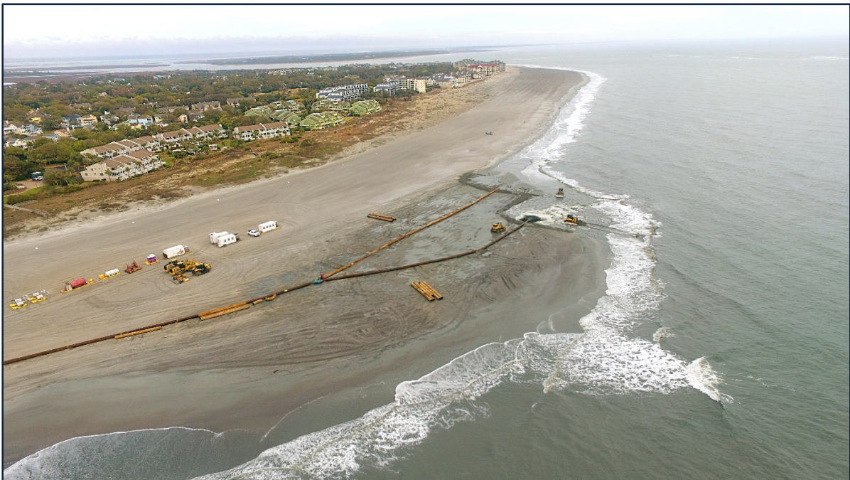
PHOTO 12. Pumping operations in front of the Beach Club Villas on 19 March 2018.
