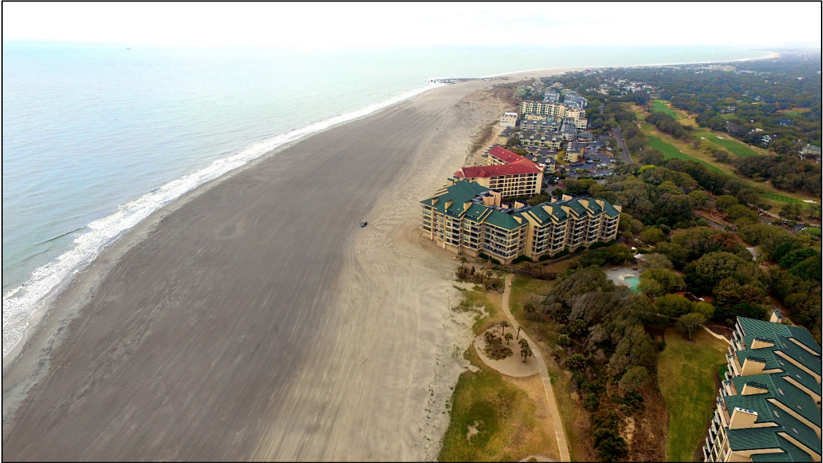
PHOTO 16. Aerial view of the north end just before project completion.
