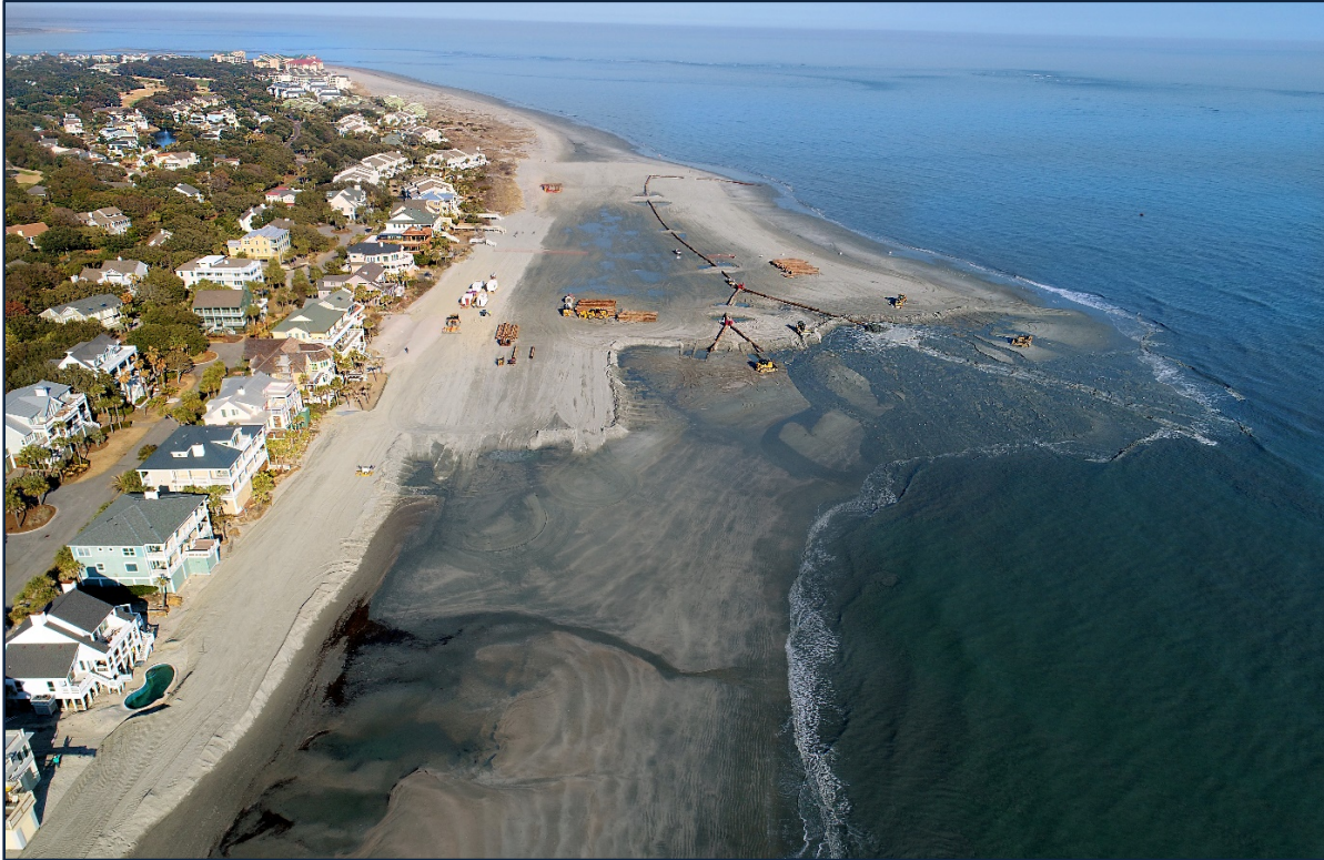
PHOTO 5. Construction progressing south in Reach 1 near Beachwood East 21 January 2019.
