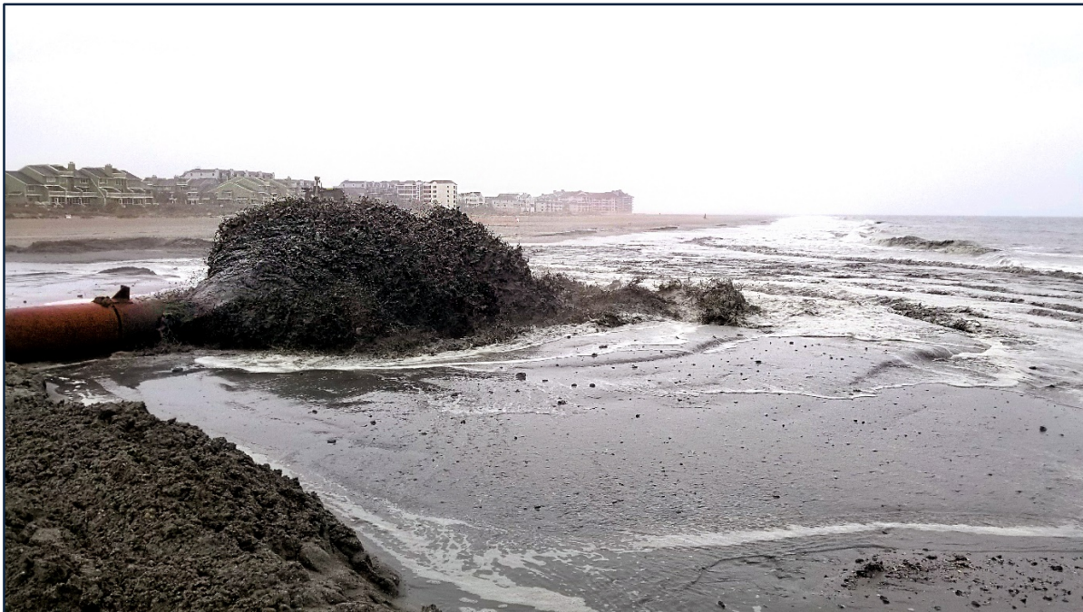
PHOTO 4. Water and Sand slurry being pumped on the beach in front of the Property Owner's Association Beach House
