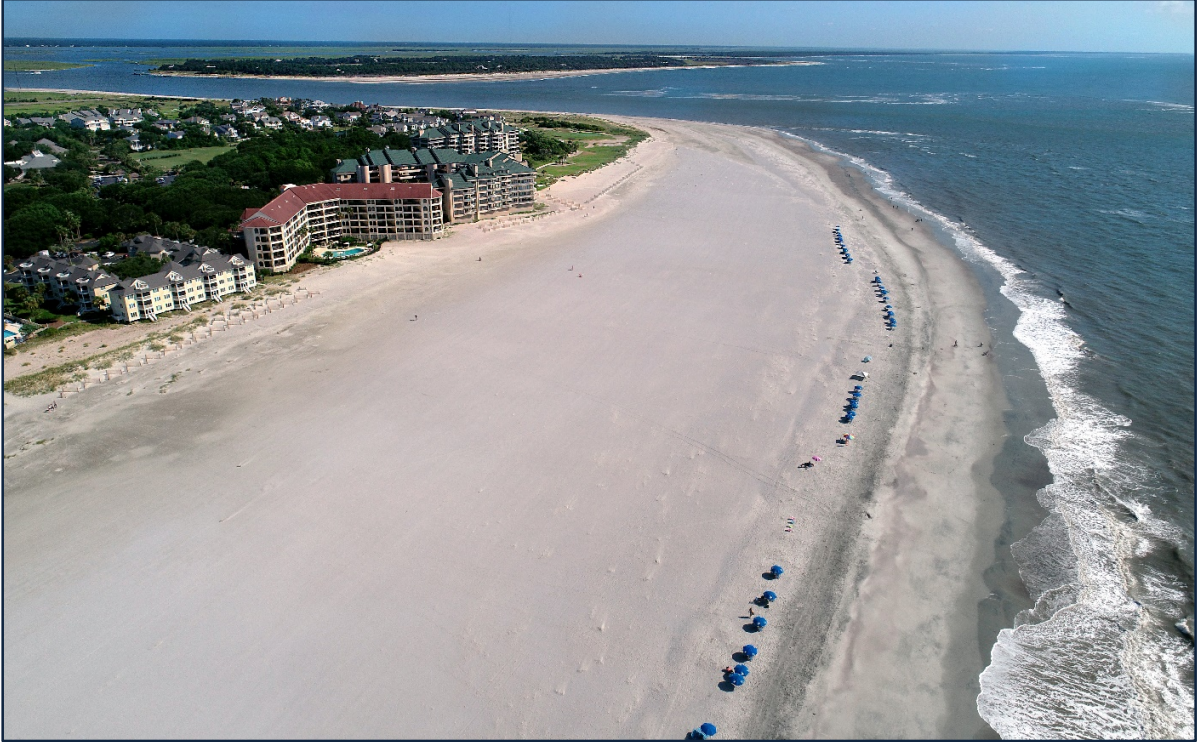
PHOTO 13. Condition of beach in front of Port O' Call, Seascape, and Ocean Club Villas almost 5 months after the project on 17 August 2018.
