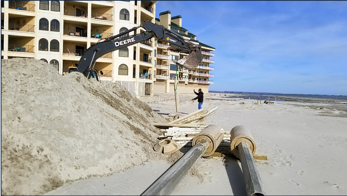
PHOTO 3. Removal of Wave Dissipation System in front of the Ocean Club Villas on 2 January 2019 prior to pumping.
