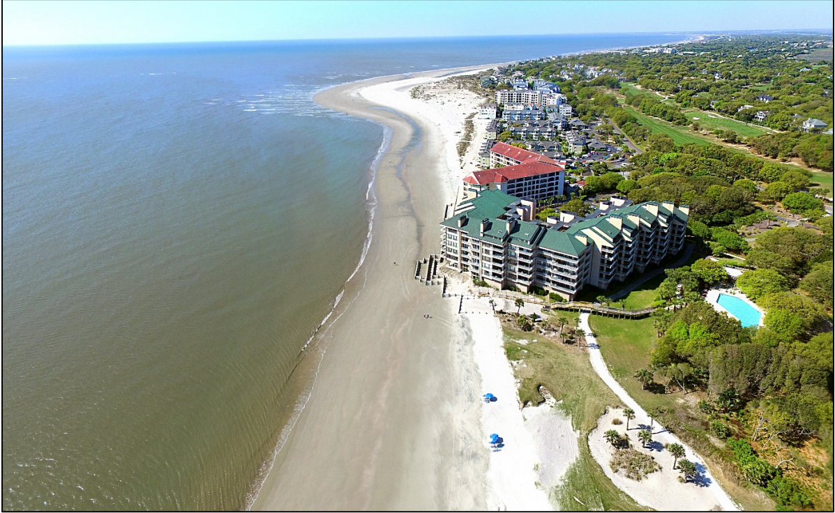
PHOTO 15. Pre-project aerial view from the north end of the island with the Ocean Club Villas and Wave Dissipation System in the forefront.
