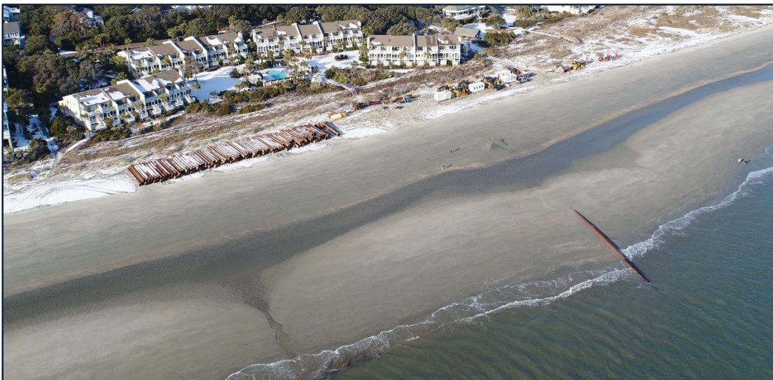
FIGURE 3.1. Initial project staging area located near Beach Club Villas. Note the rare snow event captured in the photo (date 5 January 2018).
