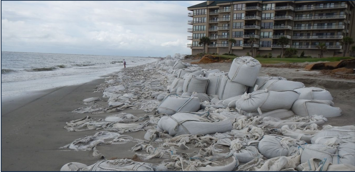
FIGURE 2.5. To prevent additional erosion, sandbags were installed along several structures from Shipwatch to Ocean Club from 2004 to 2007.
