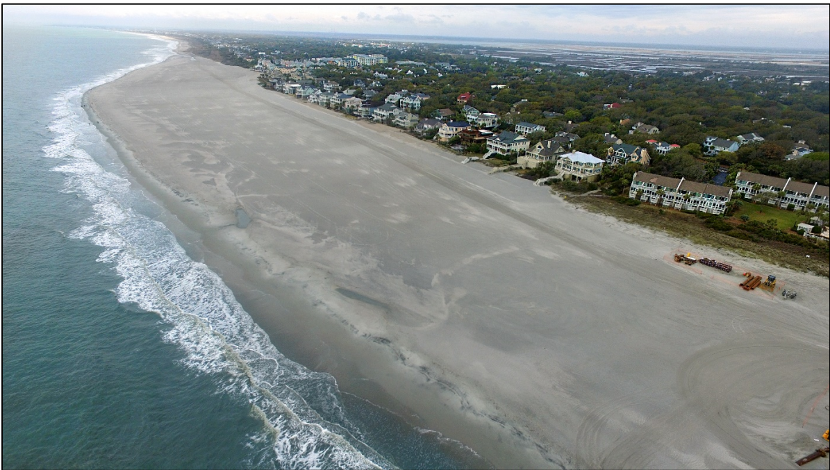
PHOTO 18. Reach 1 (Stations 236+00 through 280+00) on 19 March 2018, 4 days before project completion.
