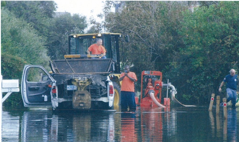
Public Works personnel pump flooded storm water
